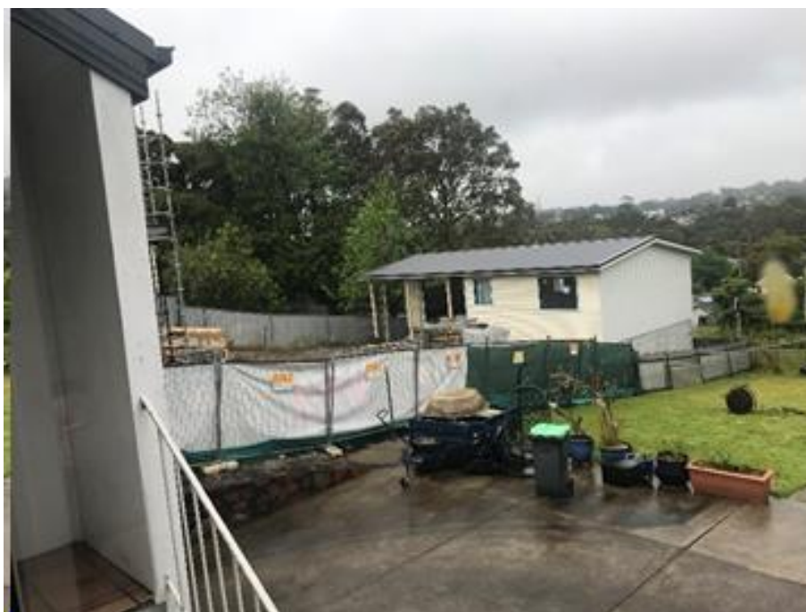
Figure 8 - Photos taken standing at windows from within Rumpus (enclosed Verandah-Living Area) of 63 Grinsell Street.
