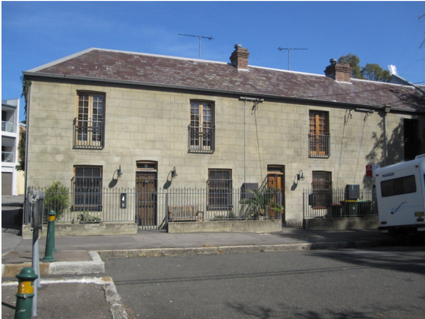
Figure 2.3 - Georgian style attached terraces on Queen Street
