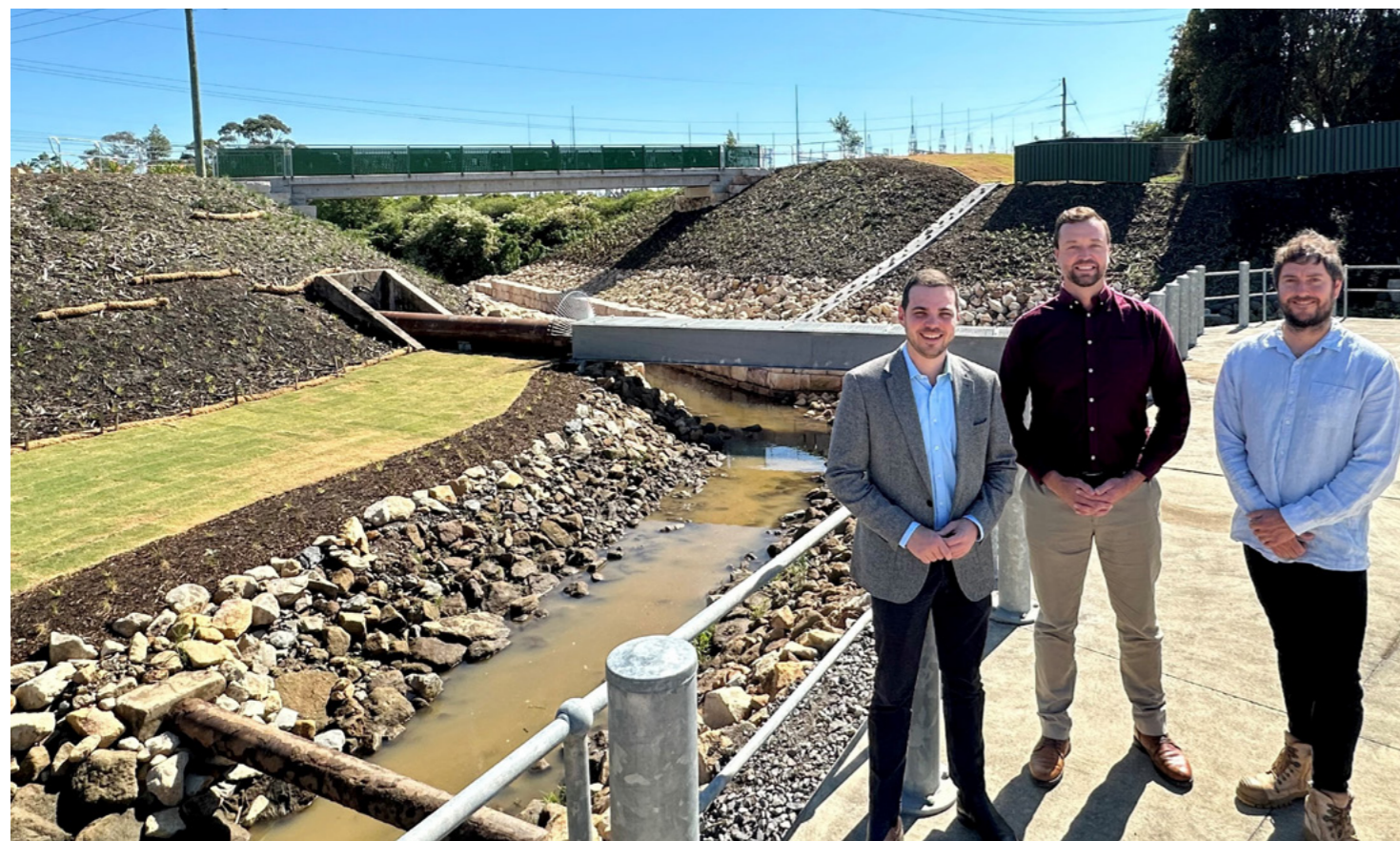
Deputy Lord Mayor Declan Clausen, City of Newcastle Assets Coordinator – Stormwater Ben Lovell and City of Newcastle Asset Engineer Luke Jaszcyk celebrate the completion of the stormwater upgrade at Boatman Creek.
