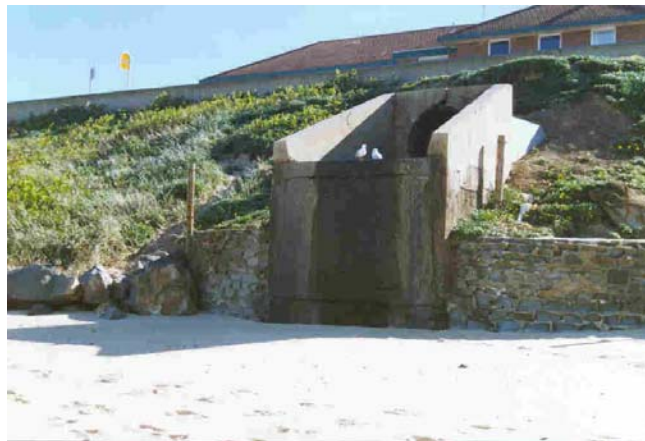
Photo 20: The headwall of the stormwater outfall at Merewether Beach
