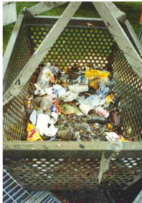
Photo 17: Shows the typical array of litter and gross pollutants removed from the trash baskets (Foreshore Park) during the regular cleaning program conducted after rain events (on average every 6 weeks).
