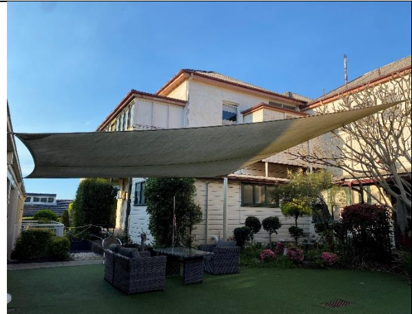
Figure 13: South-western corner of the building.
