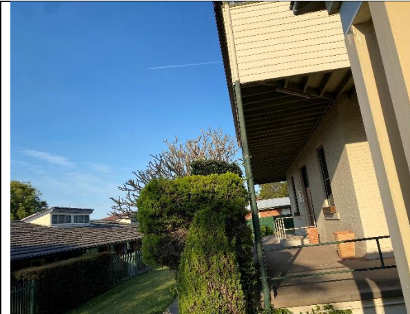
Figure 12: Oblique view of the front façade, looking east.
