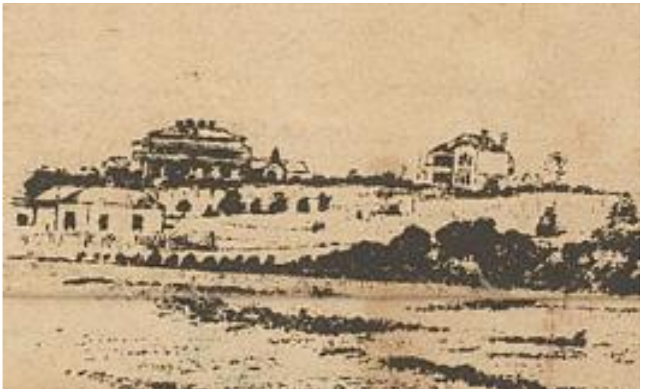
Figure 6: Extract from the above advertisement, Figure 4, depicting the subject building (left) and neighbouring residence of John Scholey (right). Both are still extant. Source: University of Newcastle Special Collections
