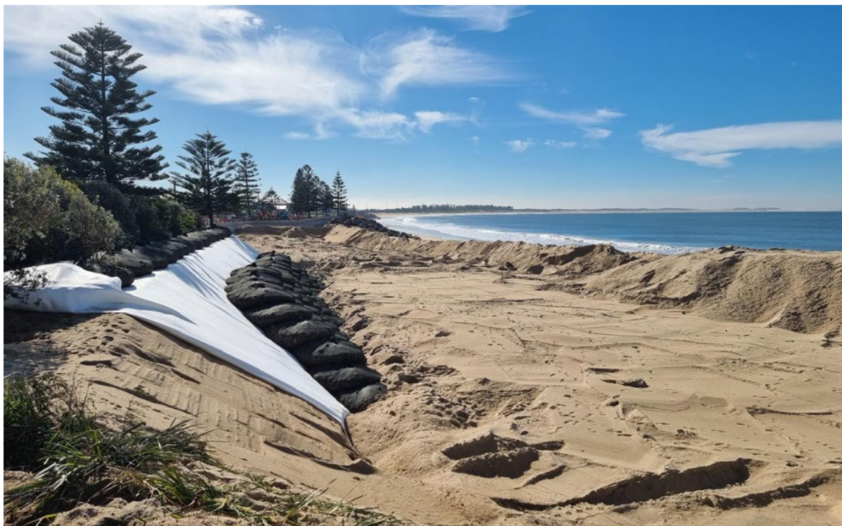
Rock bag construction. Picture supplied by Ron Boyd.
