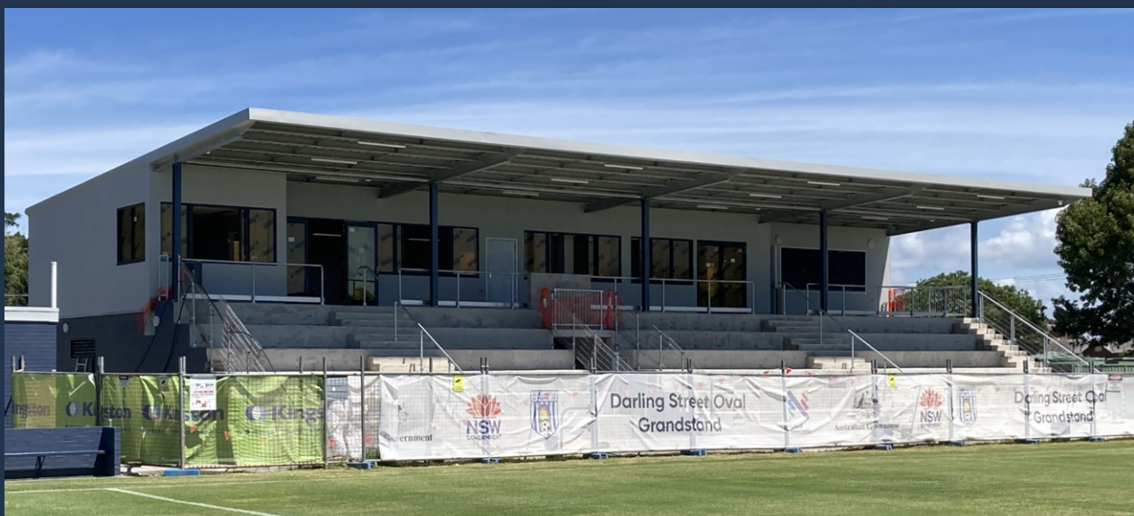
Underway: Upgrades to Darling Street Grandstand Hamilton South.
