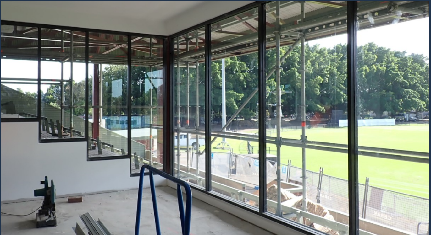
Underway: Upgrades to Passmore Oval Grandstand Wickham
