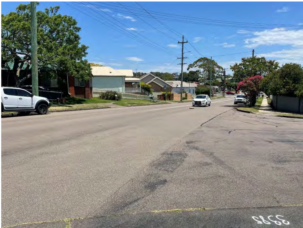
Georgetown Road / Bowker Street intersection.
