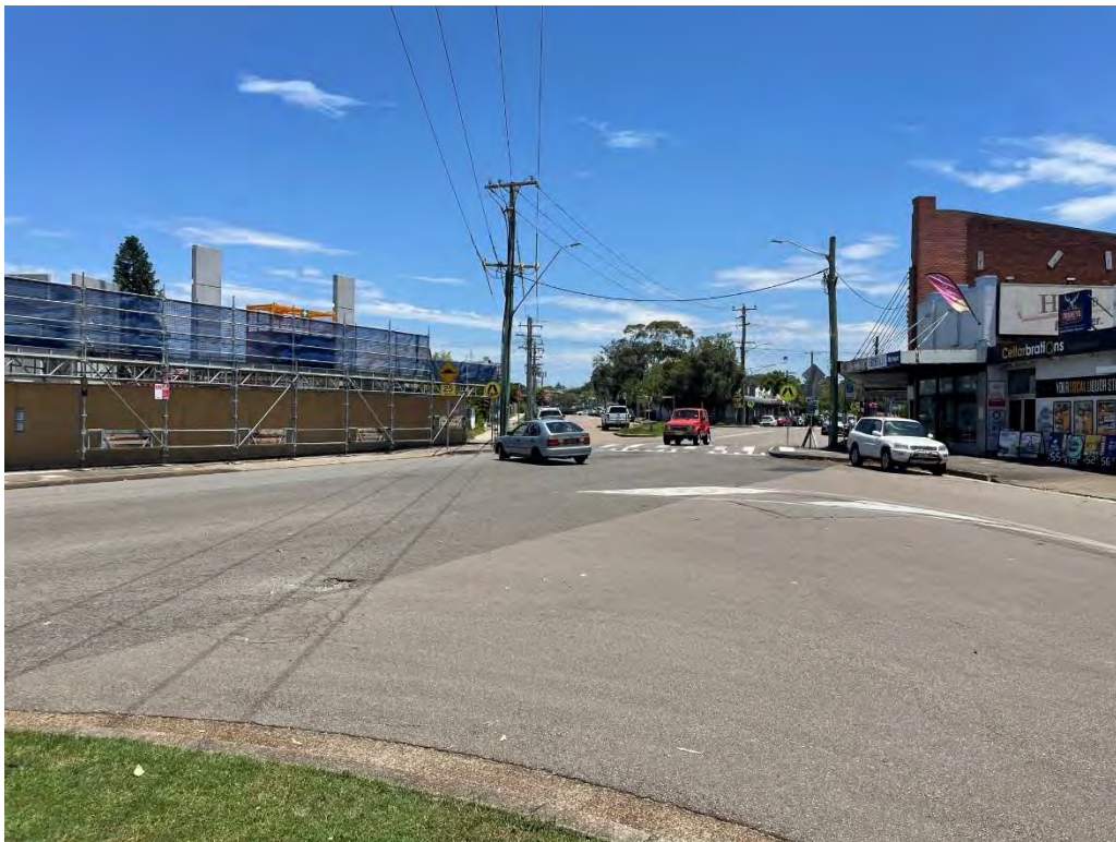
Moate Street intersection
