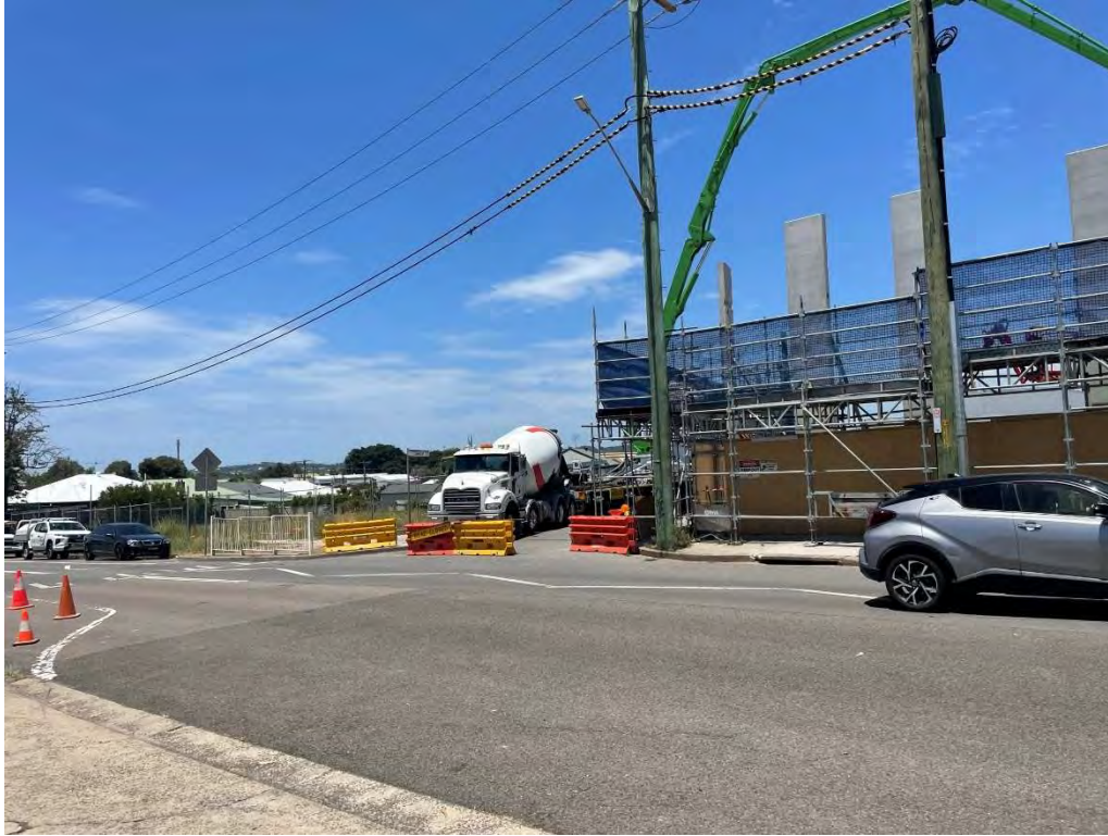
Looking towards Turner Street and construction occurring
