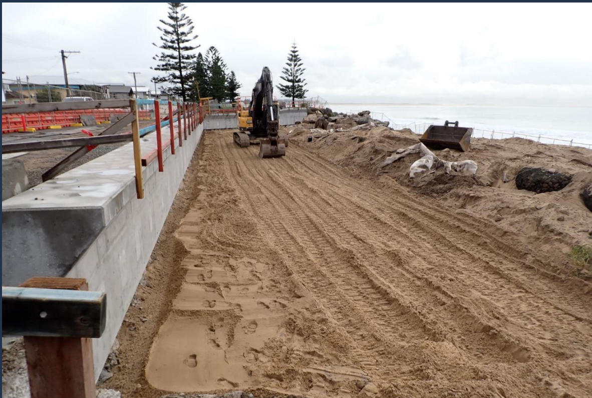
Underway: Construction of buried protection structures at Zone 2 Stockton Beach.
