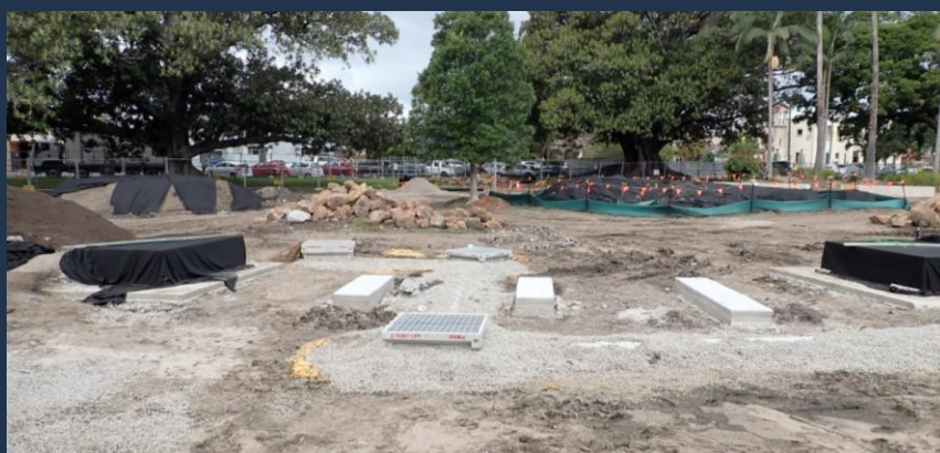
Underway: Gregson Park amenities and playground construction.
