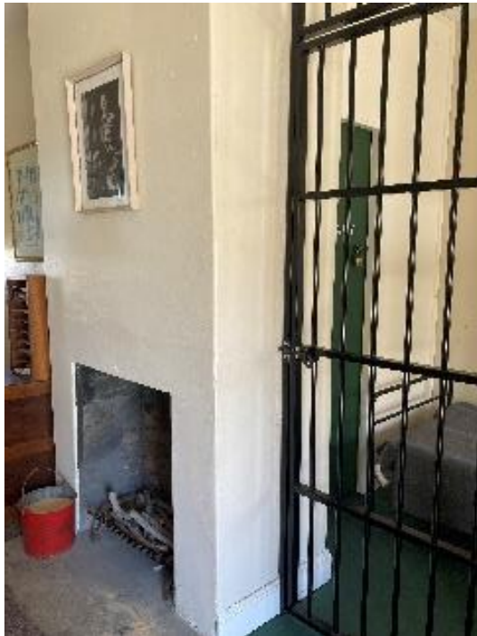
Figure 106. Interior view of Old Guardhouse, showing central fireplace and a cell. (Source: CPH, 2023)
