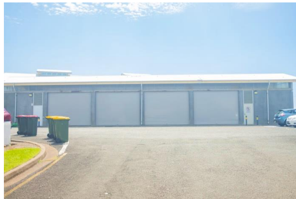
Figure 74. Workshop building, southwestern elevation. (Source: CPH, 2024)
