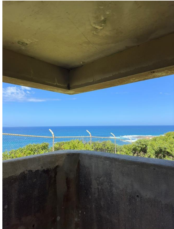
Figure 84. View towards Tasman Sea from the interior of the Searchlight Directing Station, looking southeast. (Source: CPH, 2024)
