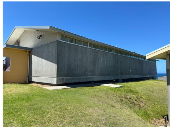
Figure 69. View of the Hall building, looking east. (Source: CPH, 2024)
