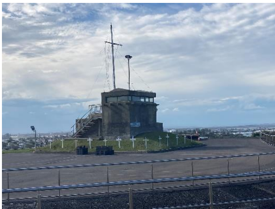
Figure 181. View to Battery Observation Post, looking north. (Source: CPH, 2023)
