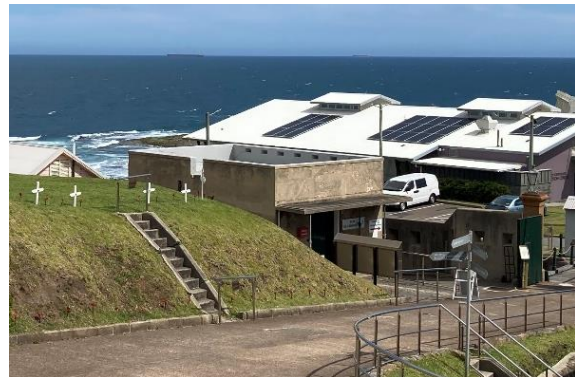
Figure 86. New Guardhouse, eastern elevation showing parapet with embrasures. (Source: CPH, 2023)
