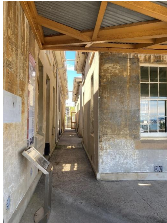
Figure 129. View towards Artillery Store (Building 15) on the right and Tunnels entrance. NCOs Quarters pictured on the left. (Source: CPH, 2023)
