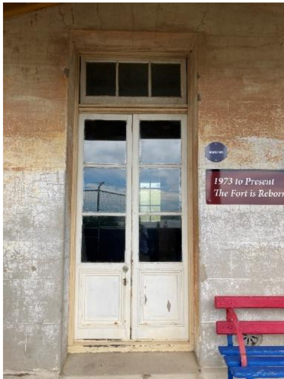
Figure 136. View of French doors with transom lights leading to northernmost bedroom. (Source: CPH, 2023)
