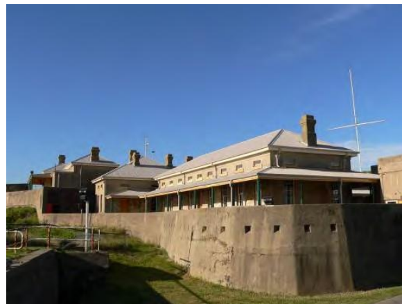
Figure 58. View of barracks complex buildings from the dry ditch. (Source: Suturs Architects, 2008)
