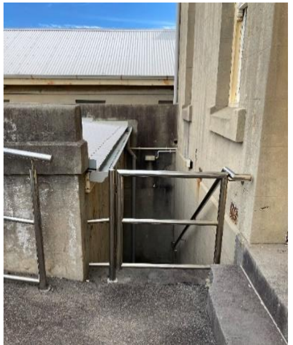
Figure 141. View of eastern steps leading to the Servant's Closet. (Source: CPH, 2023)
