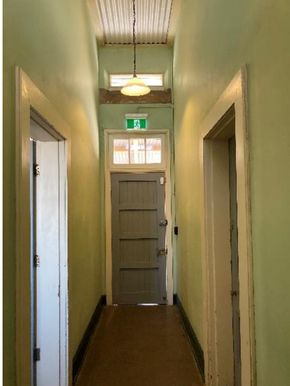
Figure 124. Internal view of the central corridor, looking east. (Source: CPH, 2023)
