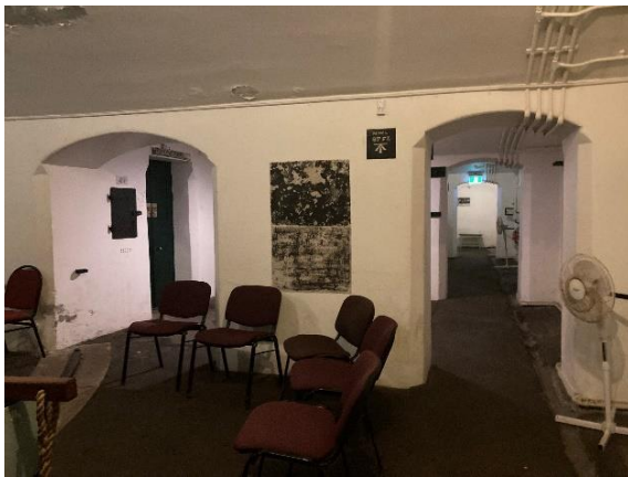
Figure 169. Internal view of Casemate Battery 2 chamber. (Source: CPH, 2023)
