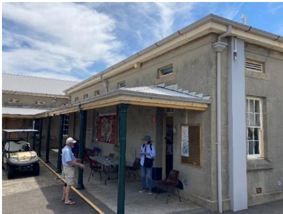
Figure 112. View of Canteen, looking north. (Source: CPH, 2023)
