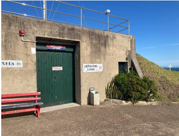
Figure 195. Exterior view of Artillery Store. (Source: CPH, 2023)
