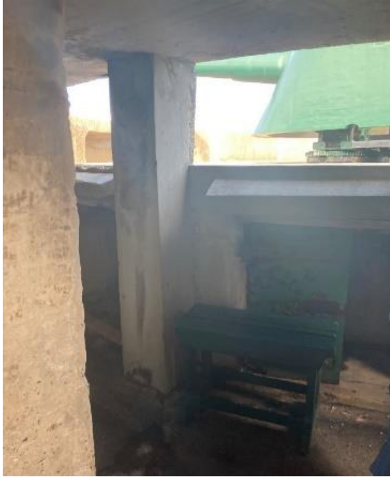
Figure 191. Stores area underneath the gun pedestals. (Source: CPH, 2023)
