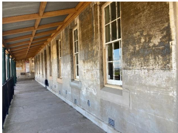
Figure 123. View of the Barracks building western façade, looking north. (Source: CPH, 2023)
