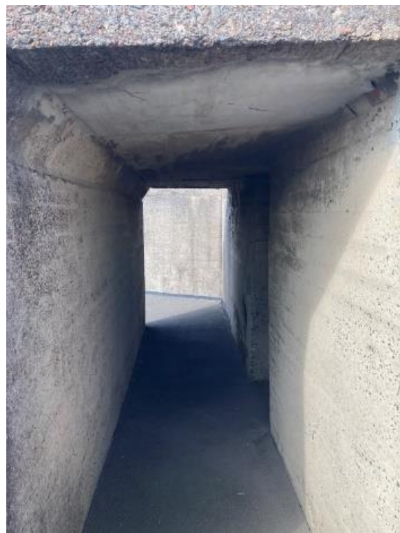
Figure 190. View of the connecting passageway between Nos. 1 and 2 Guns. (Source: CPH, 2023)
