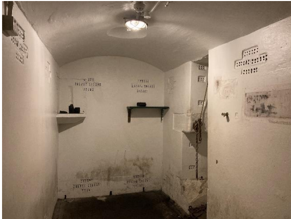
Figure 173. Internal view of ammunition lift space for Gun Emplacement 1. Note the breeze blocks and vent providing ventilation to the space. There is also evidence of original signage on the right. (Source: CPH, 2023)
