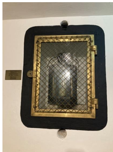
Figure 214. Restored bronze lamp recess with no visible deterioration. (Source: CPH, 2023)
