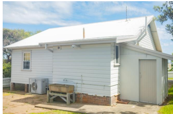
Figure 65. Master Gunner's Cottage, southern elevation, showing rear wing additions. (Source: CPH, 2024)
