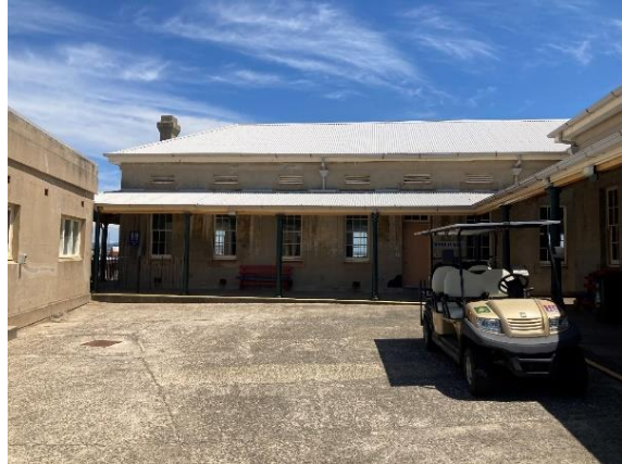
Figure 121. View of the Barracks building, looking east. (Source: CPH, 2023)
