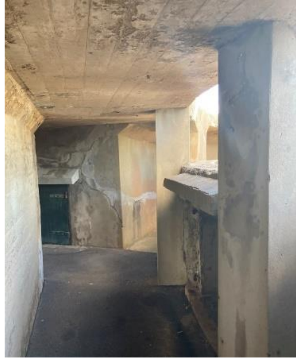
Figure 192. View of covered passageway beneath No. 1 Gun. (Source: CPH, 2023)
