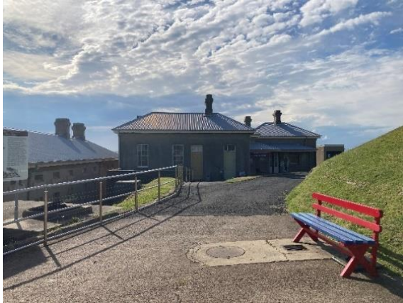
Figure 134. View towards Commandant's Cottage, looking west. (Source: CPH, 2023)
