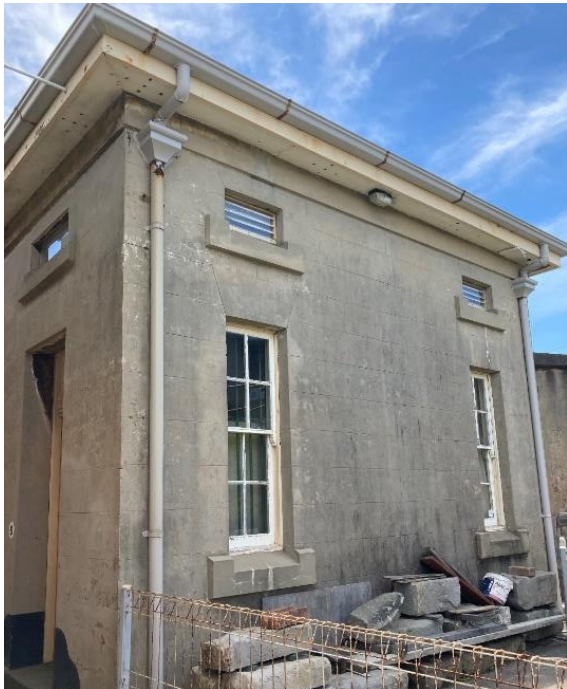
Figure 130. NCOs' Quarters, eastern elevation. (Source: CPH, 2023)
