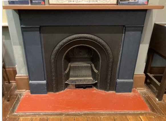
Figure 139. Reconstructed fireplace with timber mantelpiece in southern bedroom of Commandant's Cottage. (Source: CPH, 2023)
