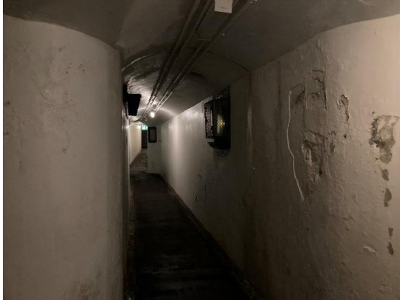
Figure 171. Internal view of tunnels leading from main magazine to the casemate batteries. (Source: CPH, 2023)
