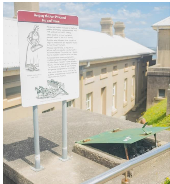
Figure 133. Top view of coal bunker. The bunker was used to store coal needed for the Fort's cooking and heating needs from 1886 until well into the 20th century. (Source: CPH, 2024)
