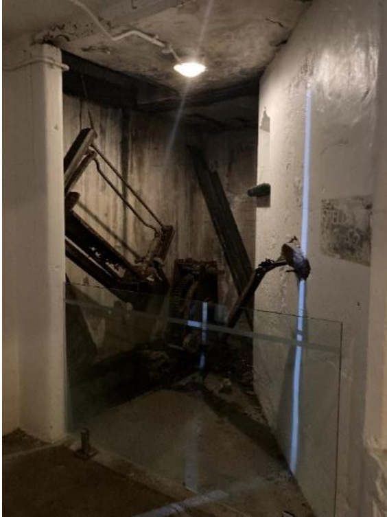
Figure 159. Example of lift machinery used to transport larger parts between levels. (Source: CPH, 2023)
