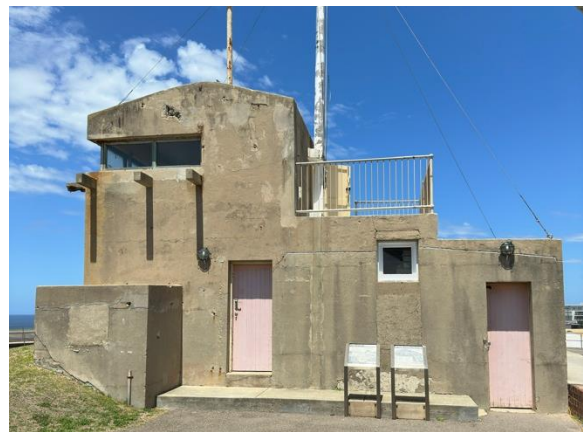
Figure 182. Battery Observation Post, northern elevation. (Source: CPH, 2024)
