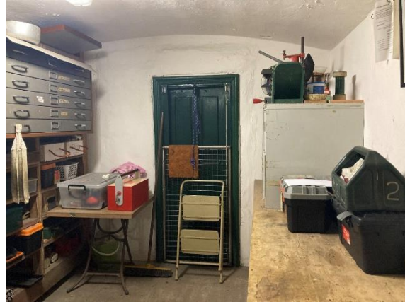
Figure 172. Internal view of eastern store room within main magazine. (Source: CPH, 2023)
