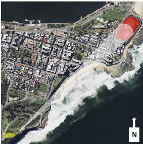
Figure 253. Views to Fort Scratchley from Shepherds Hill are possible, however, they are limited due to increasing residential development despite the higher elevation of the Shepherds Hill Defence Site. Views from Fort Scratchley to Shepherds Hill are becoming increasingly more
