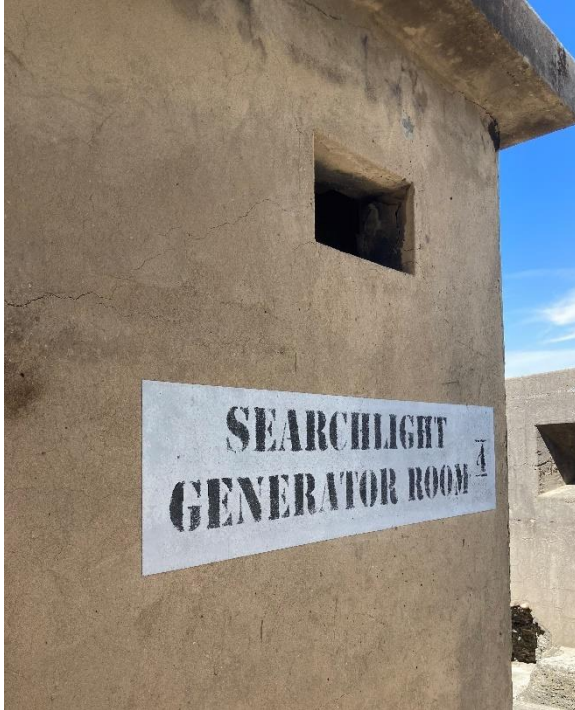
Figure 99. Searchlight Generator Room signage. (Source: CPH, 2023)
