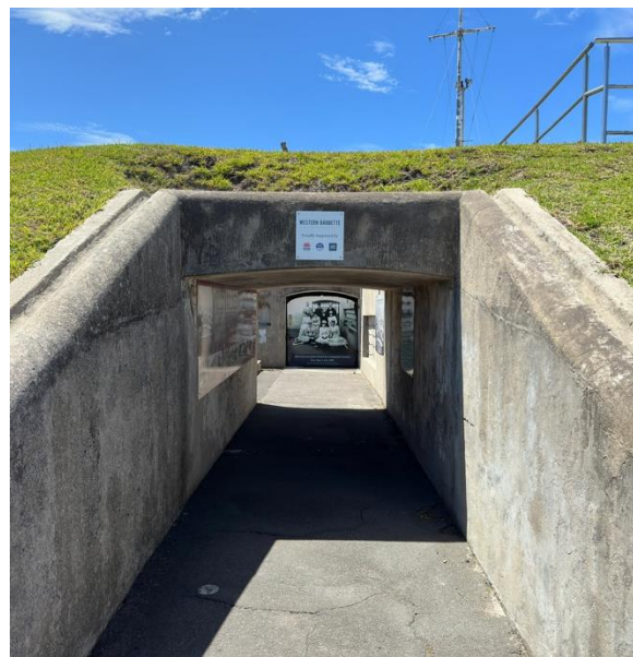
Figure 180. Entrance tunnel to Western Barbette, with interpretation panels on walls. (Source: CPH, 2024)
