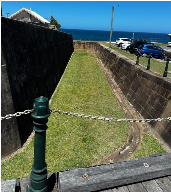
Figure 77. View of dry ditch and fortification wall, looking southeast. This section of the wall has been rendered and scored to simulate stonework (Source: CPH, 2024)
