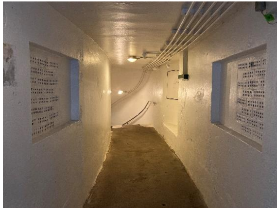
Figure 158. View to magazine level stairs. (Source: CPH, 2023)
