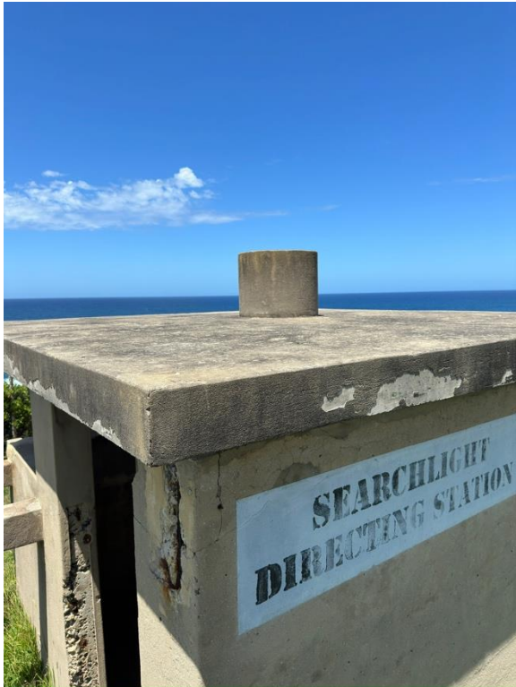
Figure 83. View of Searchlight Directing Station roof structure. (Source: CPH, 2024)
