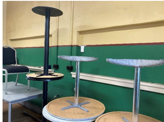
Figure 119. Internal view of the canteen room. Note the two serving hatches which have been filled. (Source: CPH, 2023)
