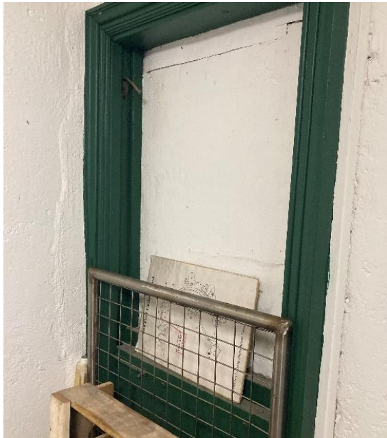
Figure 177. Evidence of previous openings in the main magazine rooms, western batching room. (Source: CPH, 2023)
