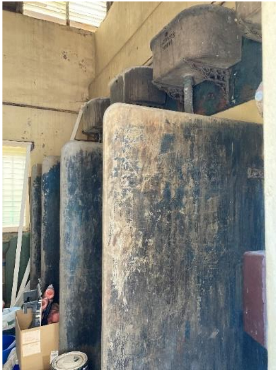
Figure 97. Interior view of the northern room. The high level cisterns remain intact. The slate partition walls are clearly visible. (Source: CPH, 2023)
