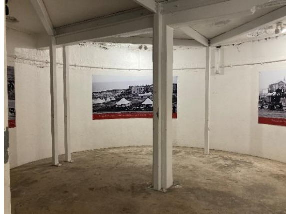
Figure 152. Internal view of Gun Emplacement 1. (Source: CPH, 2023)
