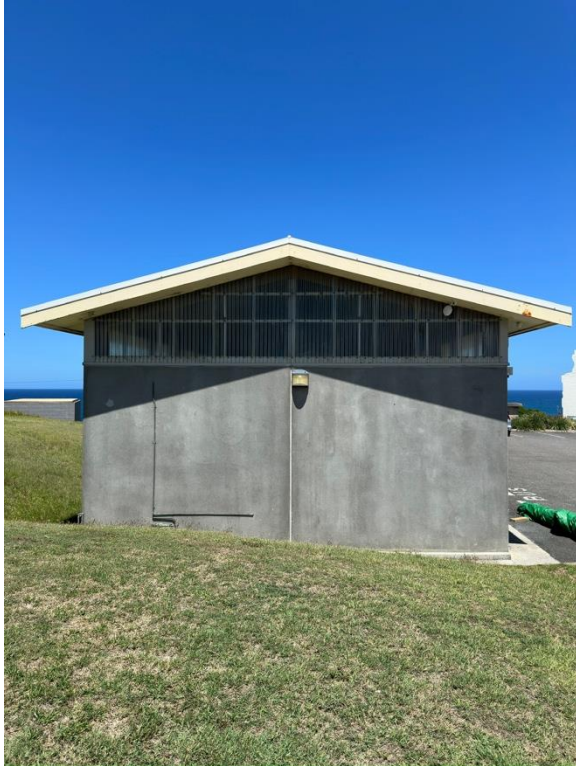
Figure 72. Workshop building, northwestern elevation. (Source: CPH, 2024)
