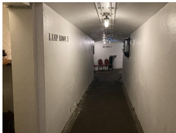
Figure 176. View of tunnel leading to magazine from southern magazine stairs. (Source: CPH, 2023)
