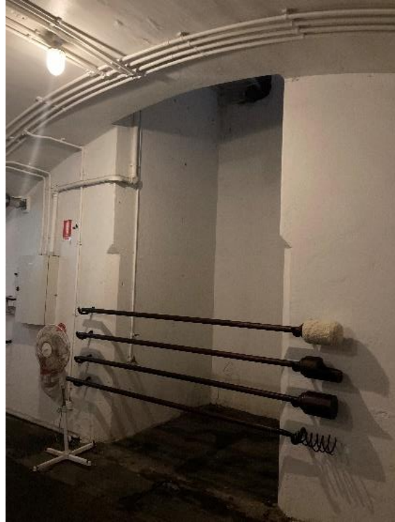
Figure 164. Ventilation shaft in Casemate Battery 2 chamber. (Source: CPH, 2023)
