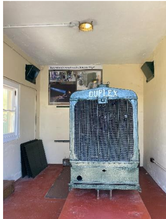
Figure 102. Interior view of Searchlight Generator Room. The generator plinth remains intact. (Source: CPH, 2023)
