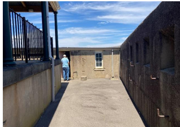
Figure 145. View towards NCOs' Ablutions, looking south. (Source: CPH, 2023)
