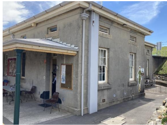
Figure 113. Canteen, eastern elevation. (Source: CPH, 2023)
