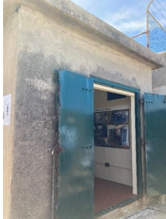
Figure 100. View of Searchlight Generator Room exterior, looking north. (Source: CPH, 2023)
