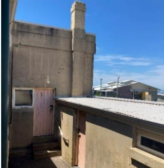
Figure 142. View of NCOs' Ablutions and Rations Block, looking east. (Source: CPH, 2023)
