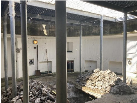
Figure 153. Internal view of Gun Emplacement 2. (Source: CPH, 2023)
