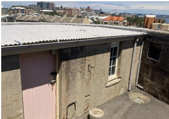
Figure 144. View over NCOs' Ablutions towards Newcastle East. (Source: CPH, 2023)
