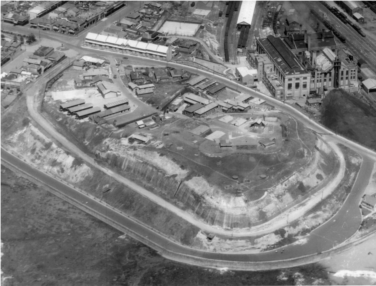
Figure 14. Aerial view of Fort Scratchley, showing additional WWII structures since demolished. (Source: Aerial photograph of Fort Scratchley with camouflage, Newcastle, NSW, 1 December 1942, R.A.A.F. University of Newcastle Library's Special Collections, FNC_402_02)
