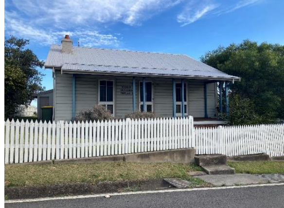
Figure 63. Master Gunner's Cottage, northern elevation. (Source: CPH, 2023)
