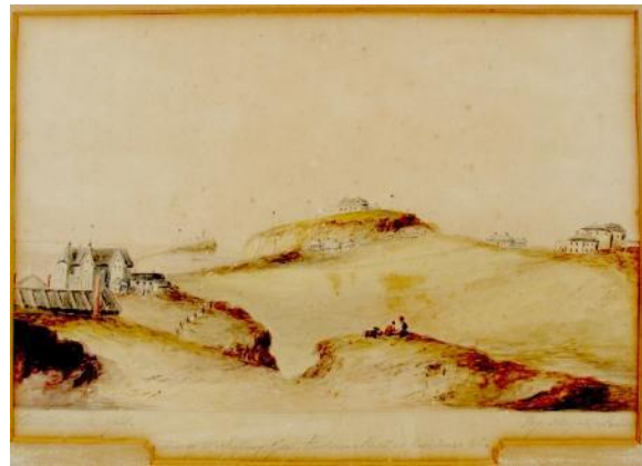
Figure 27. Sketch showing Harbour Master's residence on Signal Hill, also known as Allan's Hill after the Harbour Master. (Source: View of the infirmary, gaol, Harbour Master's residence etc sketched on the spot, c. 1870, Margaret Laidler. Newcastle Libraries, Hunter Photo Bank, 345 000256)
