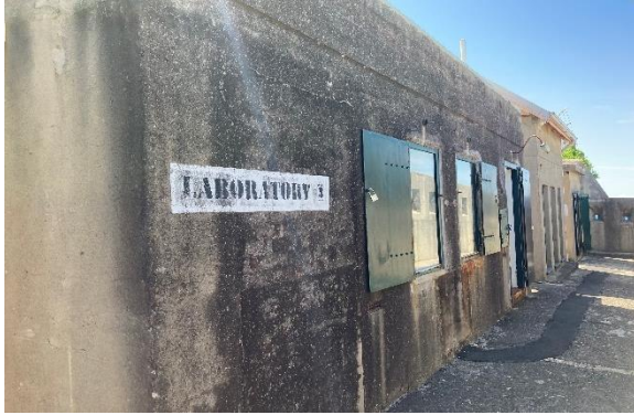
Figure 91. View of Laboratory building, looking southeast. (Source: CPH, 2023)
