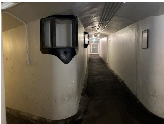
Figure 175. View of tunnel towards tunnel entrance stairs. (Source: CPH, 2023)
