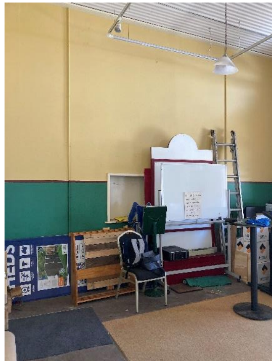
Figure 117. Internal view of the recreation room, looking east. (Source: CPH, 2023)
