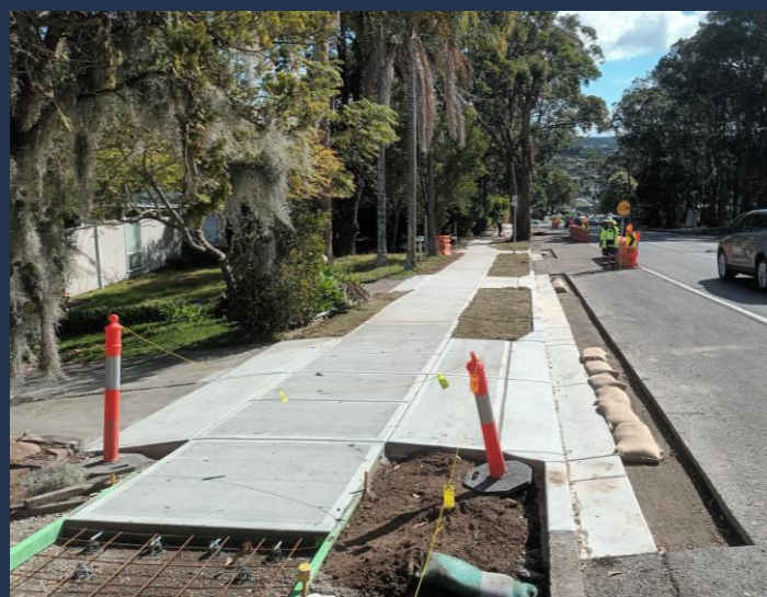
Underway: Footpath and pedestrian improvements McCaffrey Drive Rankin Park
