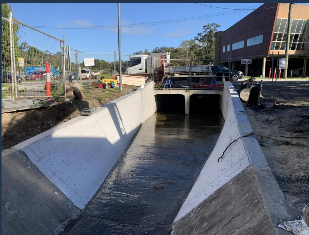
Underway: Drainage improvements at Howell Street Kotara .
