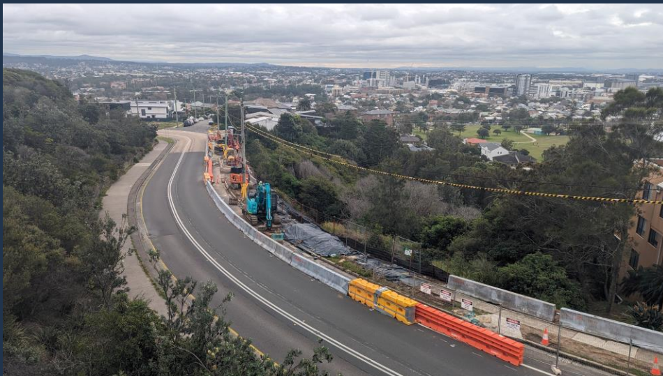
Underway: Landslip remediation at Memorial Drive The Hill .
