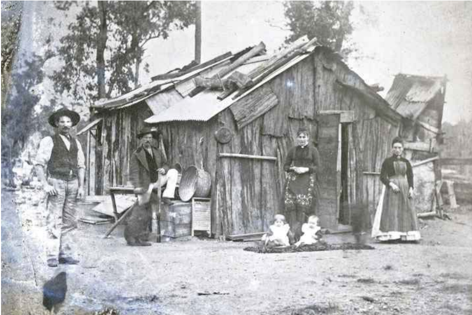
Figure 5: Typical Slab Hut, NSW (date unknown). (Source: Scanned from the original glass negative taken by Ralph Snowball. It is part of the Norm Barney Photographic Collection, held by Cultural Collections at the University of Newcastle, NSW, Australia)
