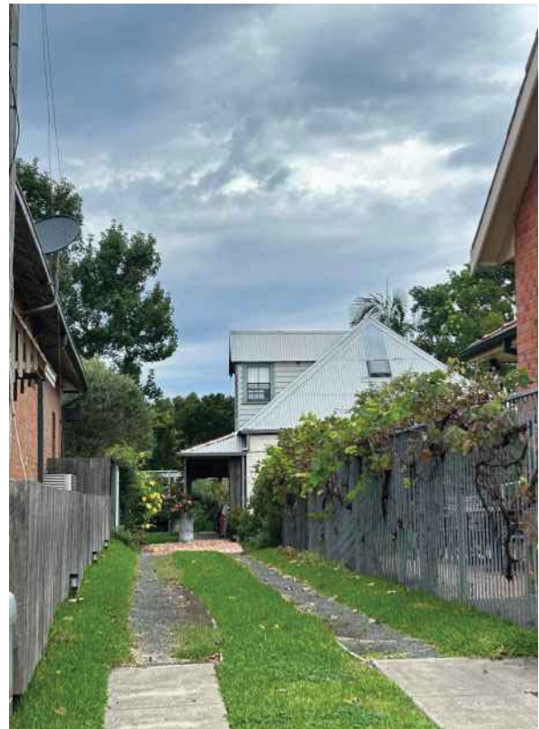
Figure 23: AA Company Mine Manager's House, Denison Street—SHR Item #01992
