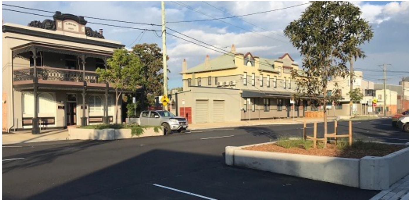
Improved drainage, vegetation and guttering in Carrington
