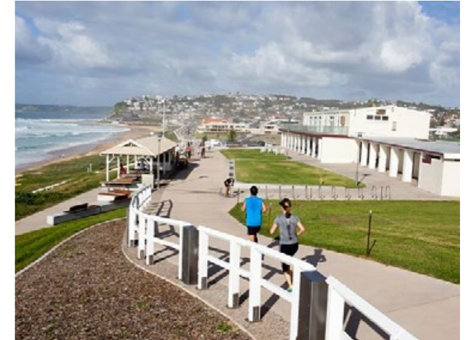
Fencing along the Newcastle Bathers way coastal walk, made from recycled wood and plastic materials
