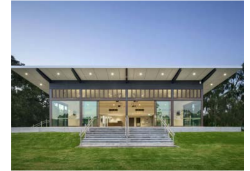
Co-located clubhouse facilities for multiple users
