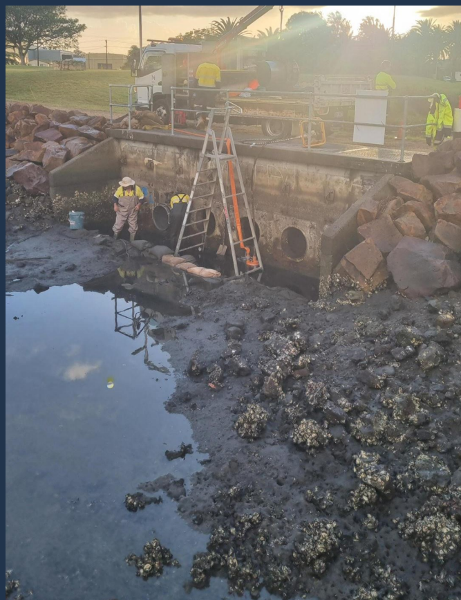
Underway: Tide gate rehabilitation Hargrave Street Carrington .
