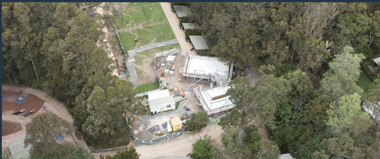
Underway: Construction of multi-purpose community facility at Blackbutt Reserve New Lambton.
